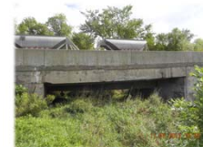
Existing Structure over Rawdon Creek
