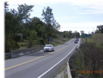
Rawdon Creek Structure (Looking South)
