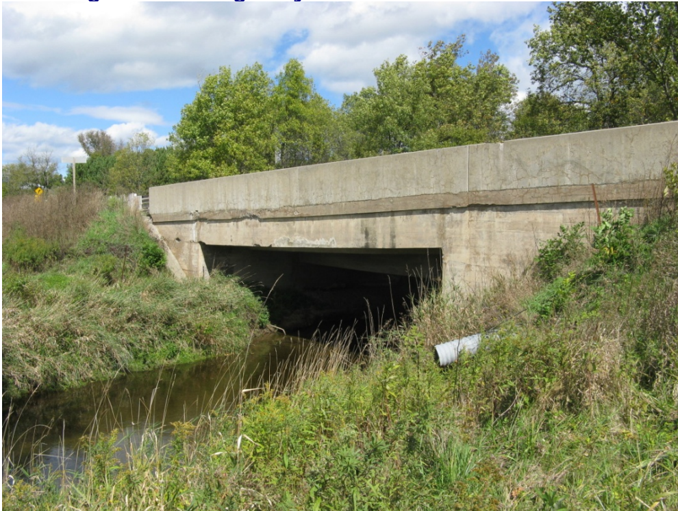
Figure 4-11: Highway 62 Rawdon Creek Structure
